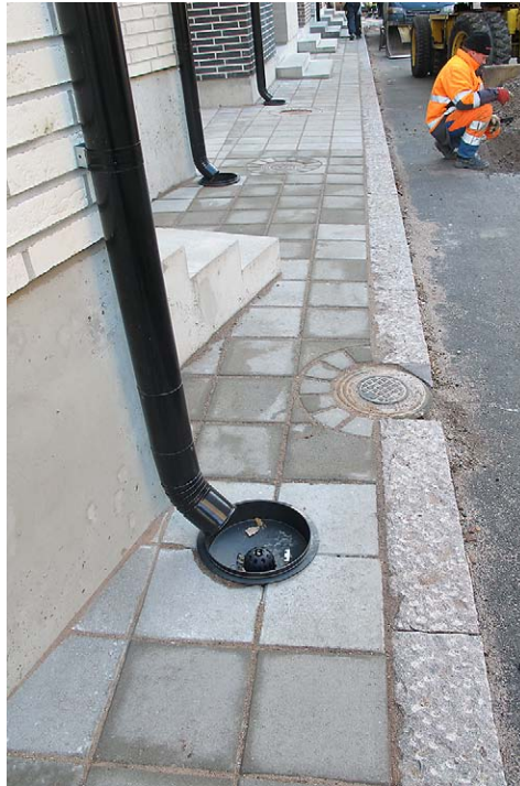
Figure 3. Incompatible design and construction of street infrastructure and housing may lead to solutions that are not accessible to any resident groups, Helsinki 2014 (photo, Verma, I.).
